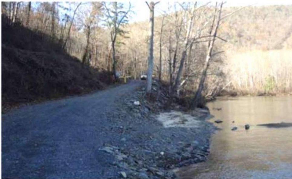
Photo 4-3: Canoe portage put-in and maintenance road accessing it from the parking area
